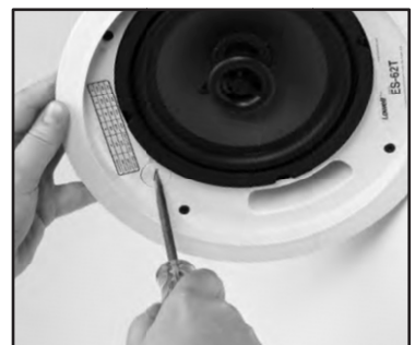
Front tap selector switch is protected behind the grille.
